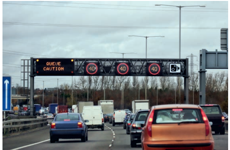
▲ Figure 5.1 Smart motorway signs
